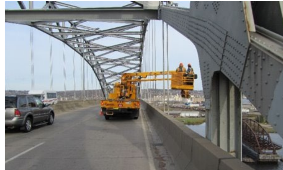
Top: Eisenhower Bridge of Valor. Bottom: Snooper truck / inspection
