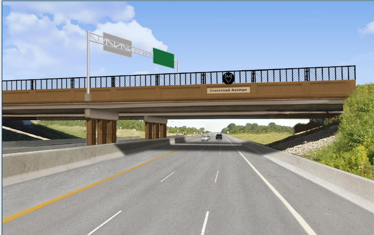
I-41 Overpass Bridge
